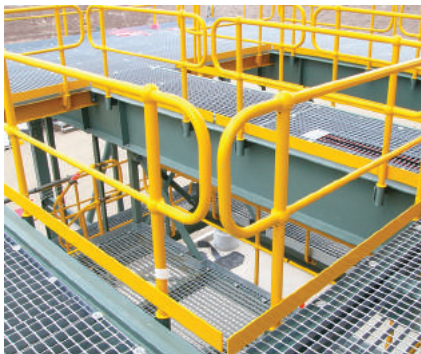
Balltube & Fabricated Handrailing
