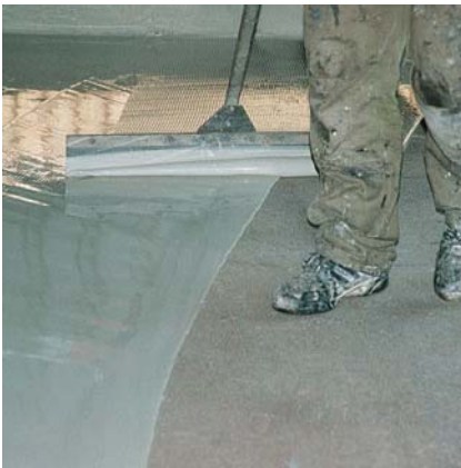
Application of a hand applied membrane.
