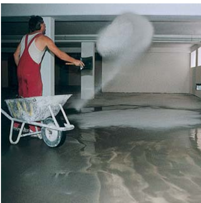
Application of primer and broadcast sand.
