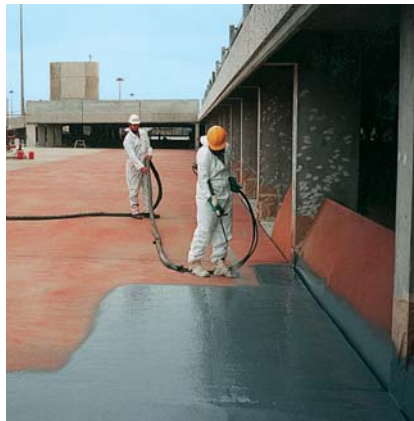
Application of the sprayed membrane.
