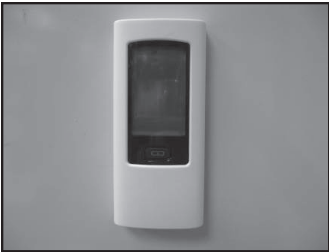
Figure 12.8 Mounting Remote Control Housing
