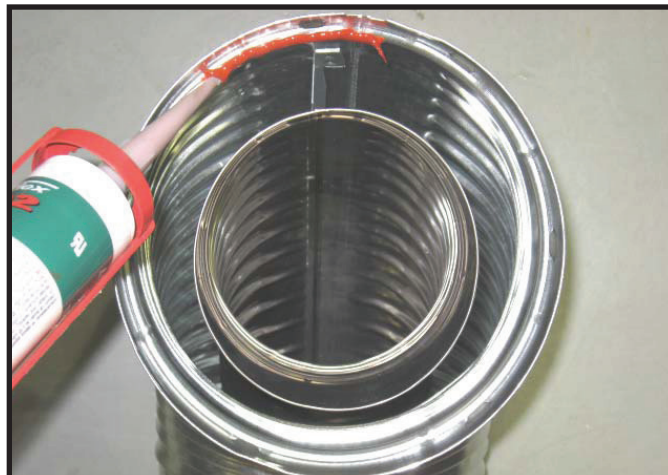
Figure 10.1 High Temperature Silicone Sealant or High Temperature Foil Tape
