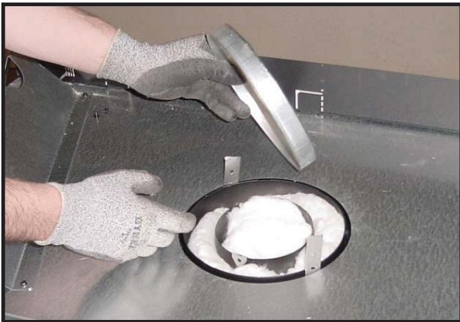
Figure 9.3 Remove the seal cap.
