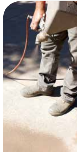
Hopper gun application of Stylepave.
