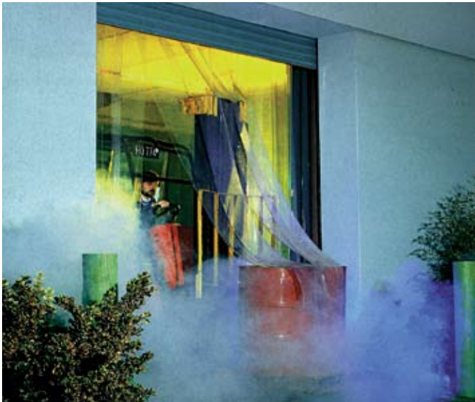
PVC Strip Door installed in Meat Processing Plant.
