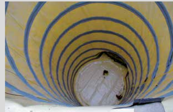
NBS Frankfurt – Köln/Germany Emergency exit shaft with Sikaplan® WT 2200-31HL2 and Waterstop MP AFI 600/35
