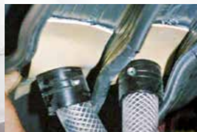
High flexible FPO membranes allow to weld difficult sections of tunnels without cutting.
