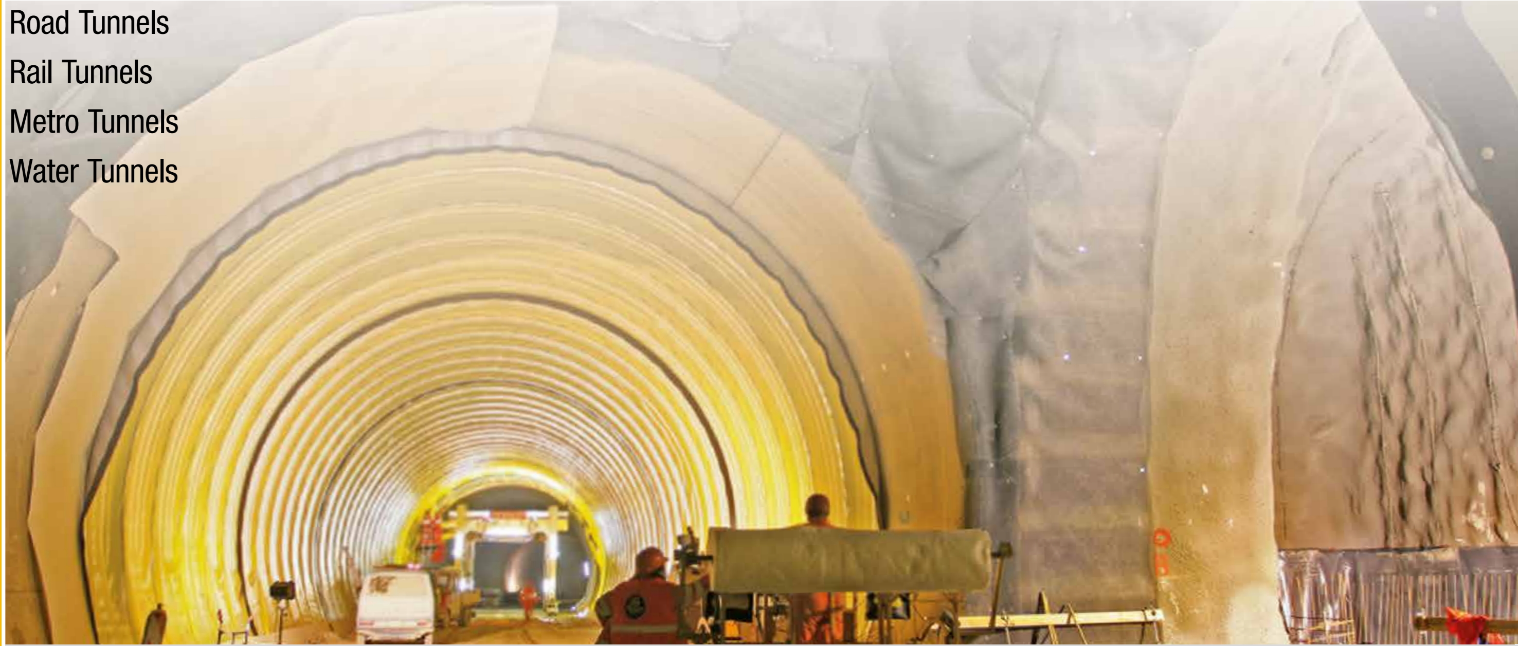
Islisberg/Switzerland, TBM construction with Sikaplan® WP 2110-20HL and fixing with hot-meld
