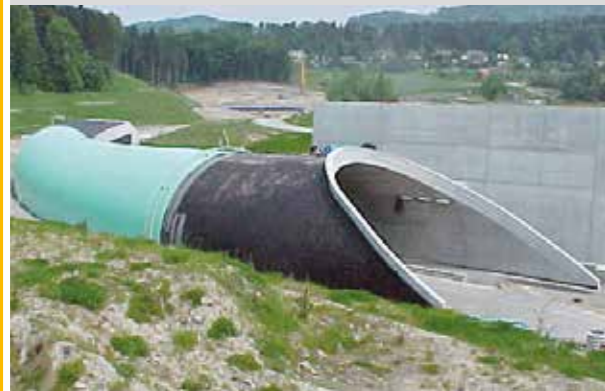
Birmensdorf/Switzerland Open cut construction with Sikaplan® WT 1200-30C
