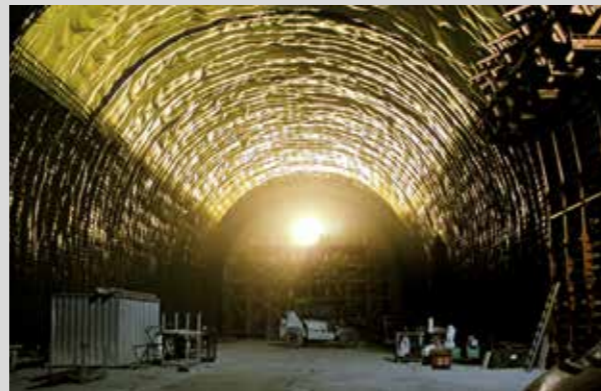
Lötschberg/Switzerland Drill and blast construction with Sikaplan® 14.6 NEAT
