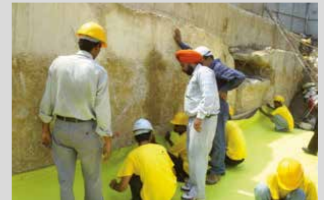
DMRC/India Open cut construction with Sikaplan® WP 1100-20HL
