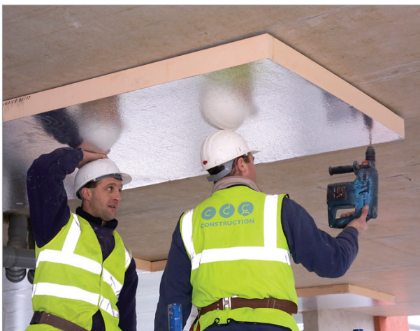
Figure 7. Penetration example - Kingspan Kooltherm® K10 G2W White Soffit Board installed tight around the fire collar and HDPE service pipe.
