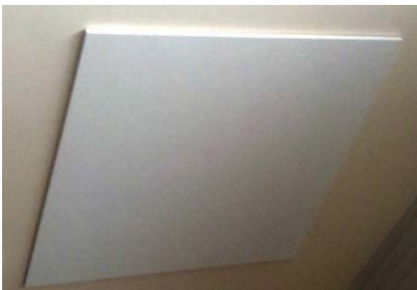
Sonofonic Square Edge Panels installed using direct fix method
