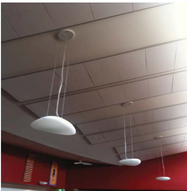
Sonofonic Square Edge Panels fixed directly to the ceiling, and with a perimeter C Channel moulding covering the exposed edge.
