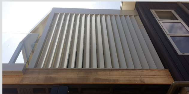
165MM HI-SPAN BALUSTRADE ALUMINIUM FRAME, VERTICAL PANEL
