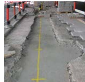
Shallow mount footings require minimal excavation and concrete.
