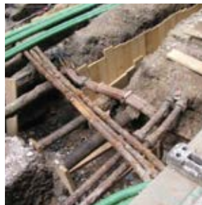
Underground services that prohibit the installation of traditional deep footings.
