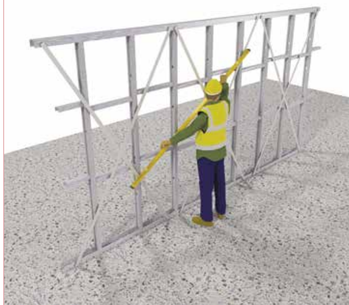
FIGURE 7 / FRAME STRAIGHTNESS
