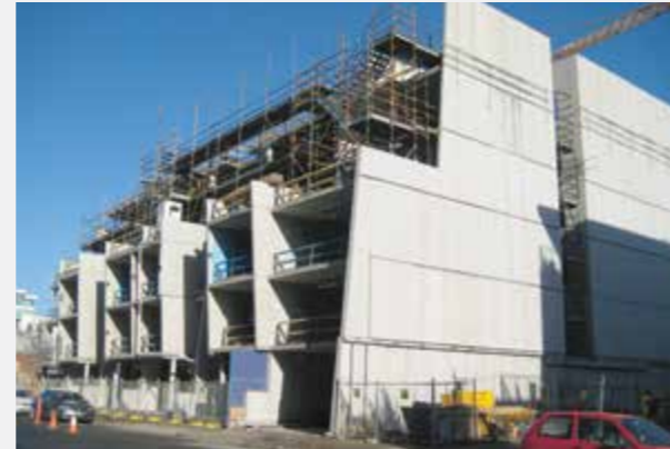
external façade walls in construction
