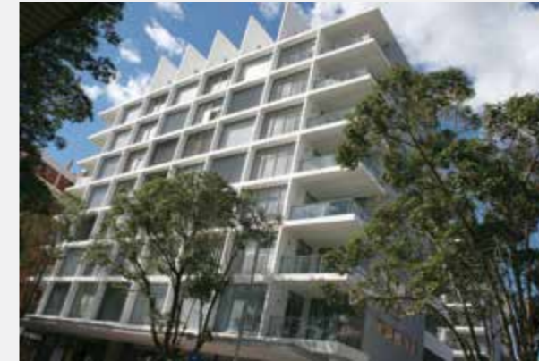
external blade walls
