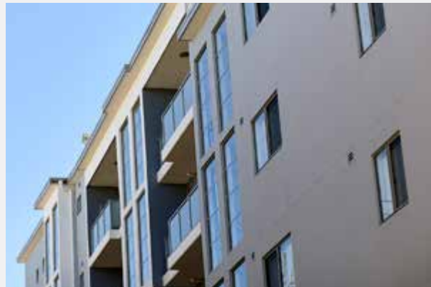
external façade walls
