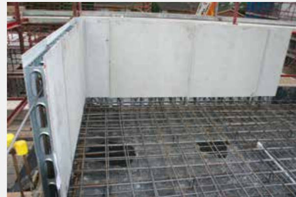
balustrade in construction
