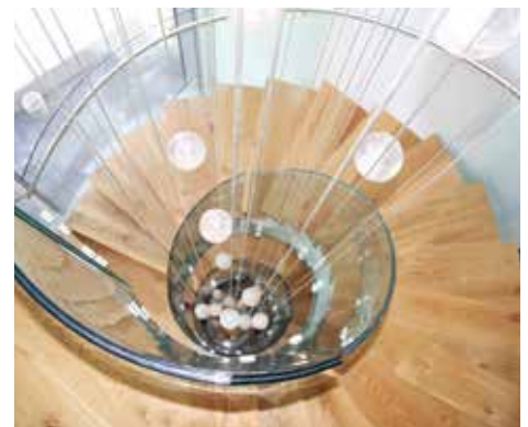
Inner balustrade: 15.04mm clear toughened structural laminated curved glass Engineered for compliance without handrail
