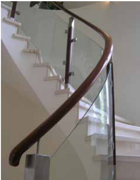
10mm clear toughened & 11mm clear laminated curved glass cantilever frameless stair panels
