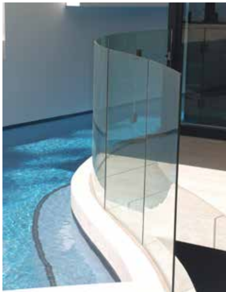
12mm clear toughened curved glass frameless, Non shrink grout fixing into concrete slab
