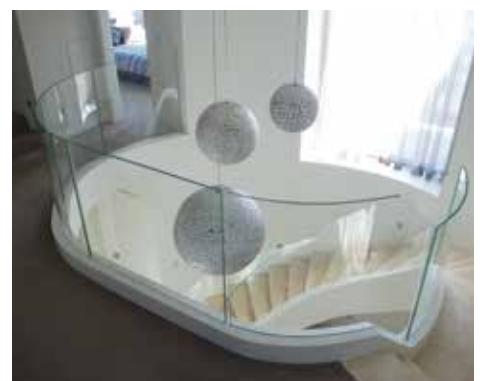
15.04mm Starphine toughened structural laminated curved glass balustrade. Engineered for compliance without a top rail
