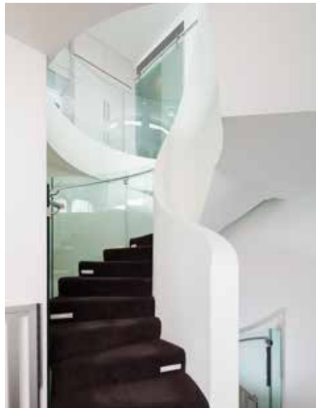
12mm clear toughened curved glass stair balustrade
