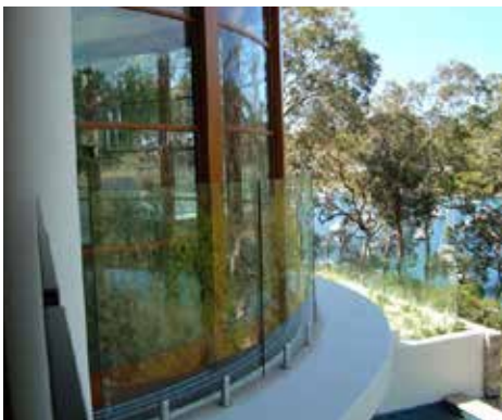
12mm clear toughened curved glass balustrade
