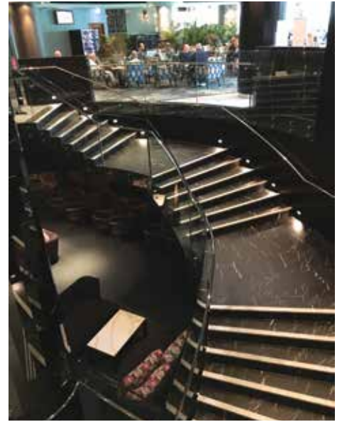
25.25mm toughened laminated curved glass balustrade
