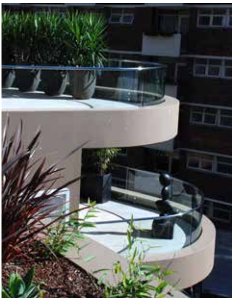
12mm clear toughened curved glass sided fixed balustrade
