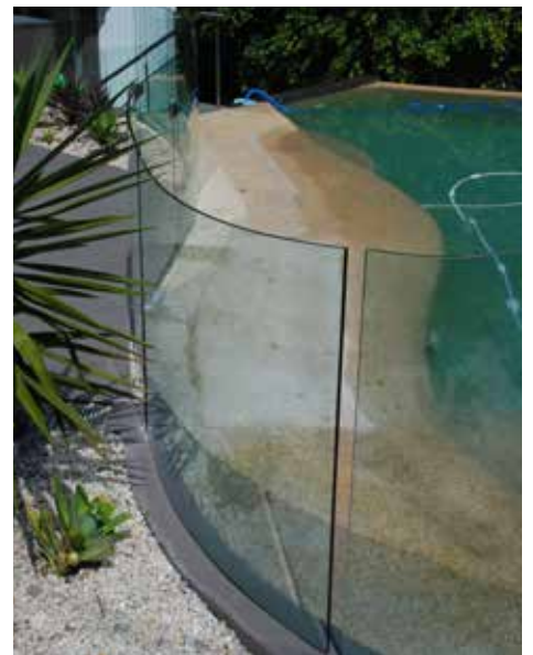
12mm clear shapecut toughened curved. Non shrink grout fixing into rebate in concrete retaining wall
