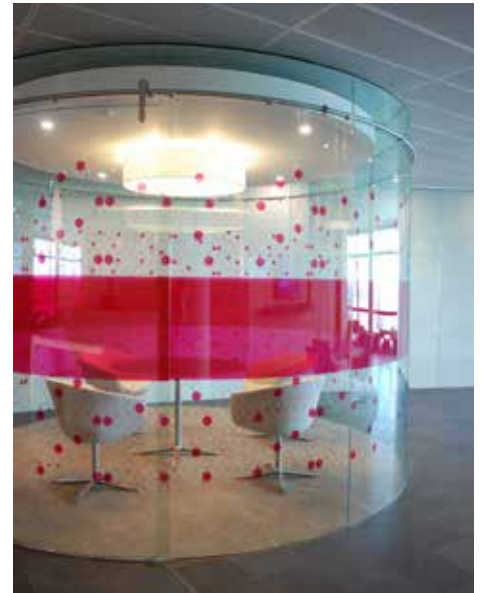
12mm clear toughened curved glass with applied decorative film Office meeting room
