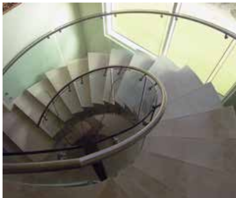
12mm clear toughened curved glass panels cantilever frameless panels with standoff patch fittings
