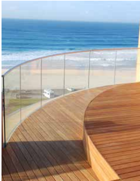
15mm clear toughened heat soaked curved glass balustrade
