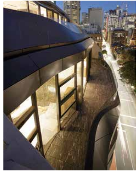
15.04mm clear toughened structural laminated curved and flat glass balustrade Engineered for compliance without a top rail
