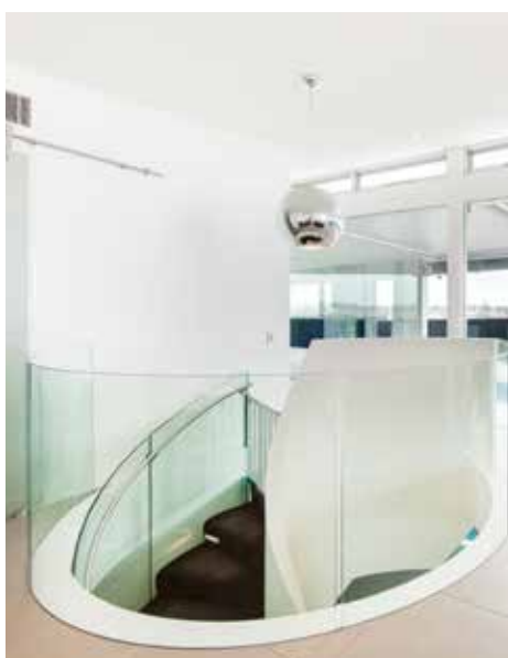
15.04mm clear toughened structural laminated curved glass balustrade Engineered for compliance without a top rail
