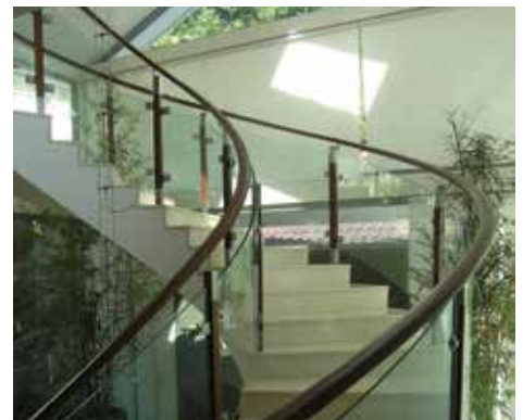
12mm clear toughened curved glass stair balustrade panels cantilever frameless panels with standoff fittings
