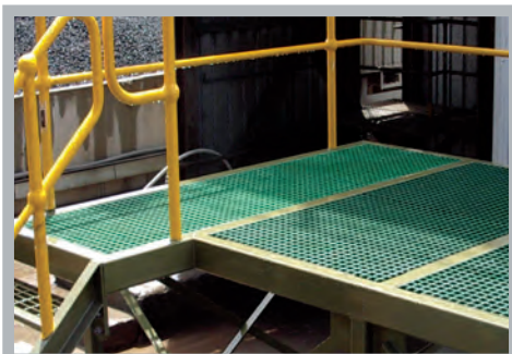
Concrete batching plant, Busselton, WA
