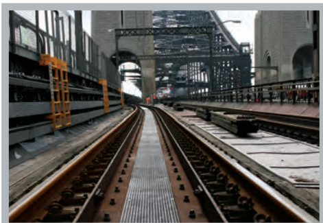
Sydney Harbour Bridge rail walkway
