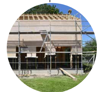
Construction panels for thermal insulation
