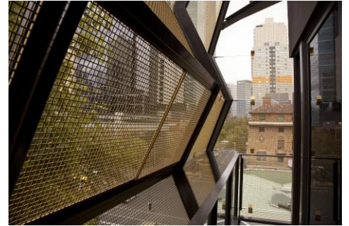
* Typical Architectural Installation
