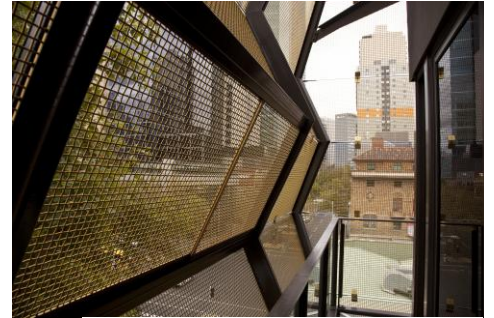
* Typical Architectural Installation
