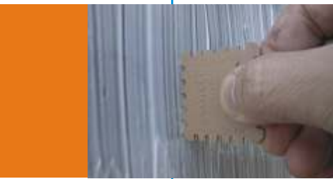
Measurement of applied film Thickness
