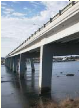
Phillip Island Bridge, Victoria Australia
