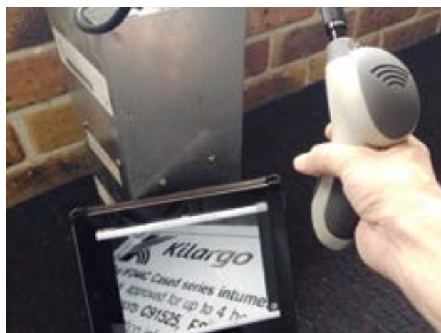
Remote visual inspection camera for maintenance inspections of intumescent fire dampers.
