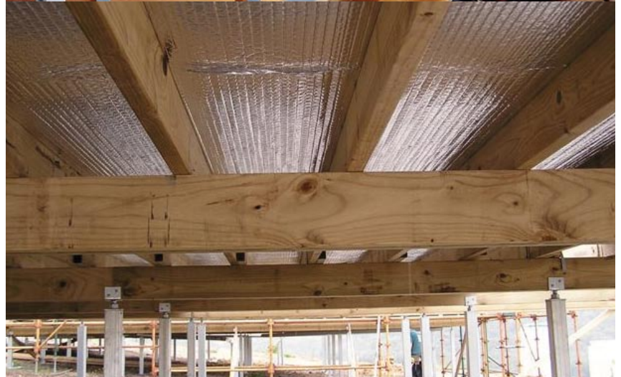
AIR-CELL® Insulation recommends installation over bearers. Please check requirements with your local council. While the above images show AIR-CELL Glareshield® installations, Permifloor™ is installed in the same manner.
