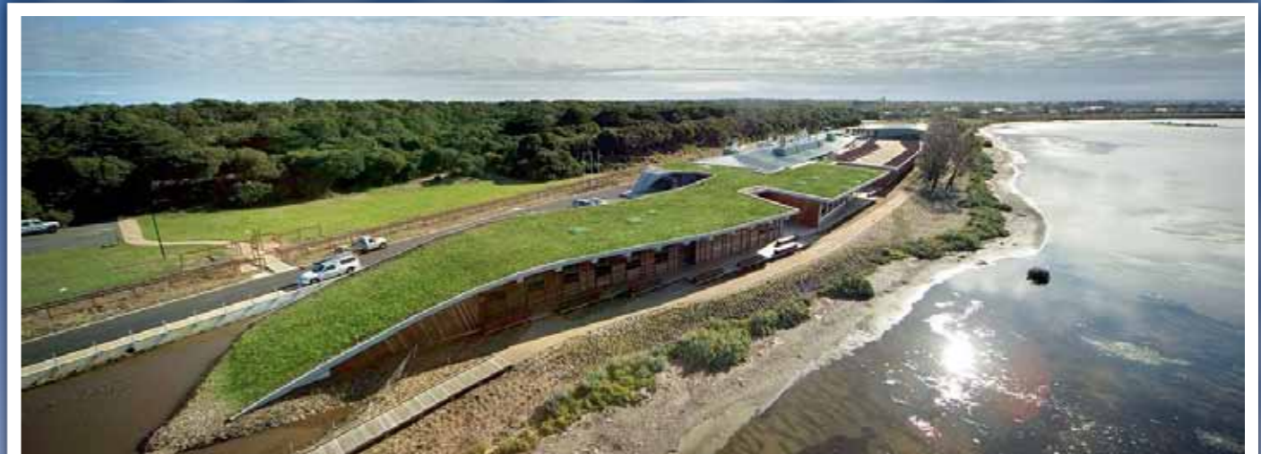
Atlantis drainage layer was installed into the roof of the Marine Discovery Centre, Queenscliff, VIC
