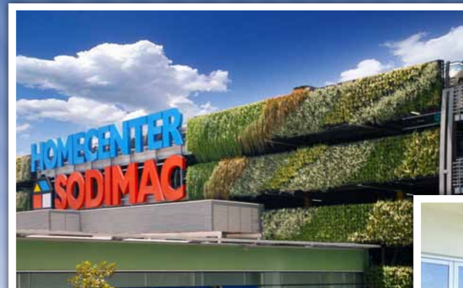
Atlantis green wall installation onto multilevel car parking, Santiago, Chile.
