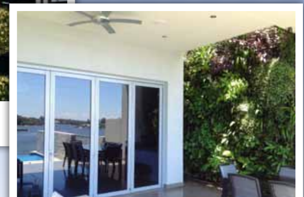
Atlantis green wall installation a residence, Sydney, Australia.
