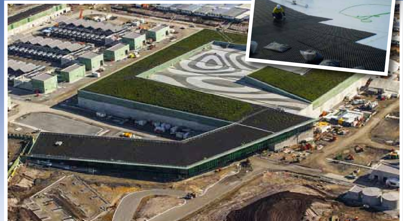
The largest roof garden in the Southern Hemisphere, 27,000m 2 . Atlantis 20mm Flo-Cell® was used as a drainage layer on the roof top garden.
