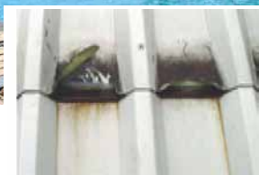
Standard plastisol on hot dip galvanised steel substrate roof after 7 years.
