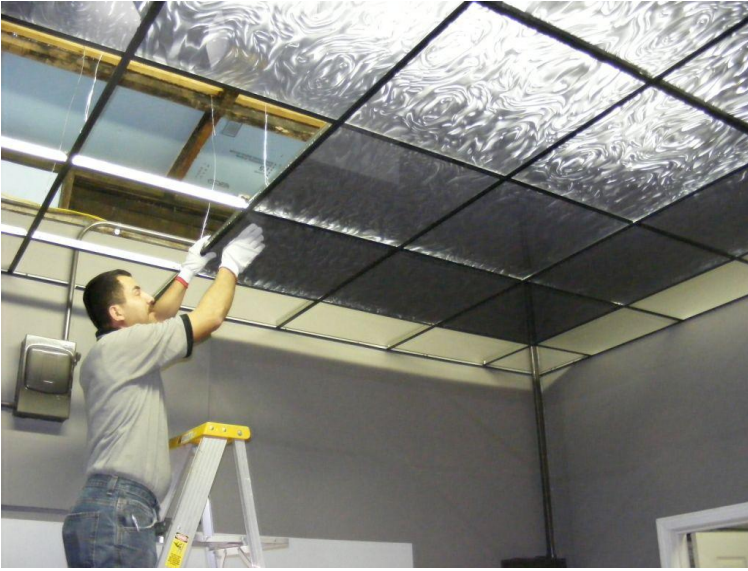
Rowlux - Ceiling Tiles - Installation
