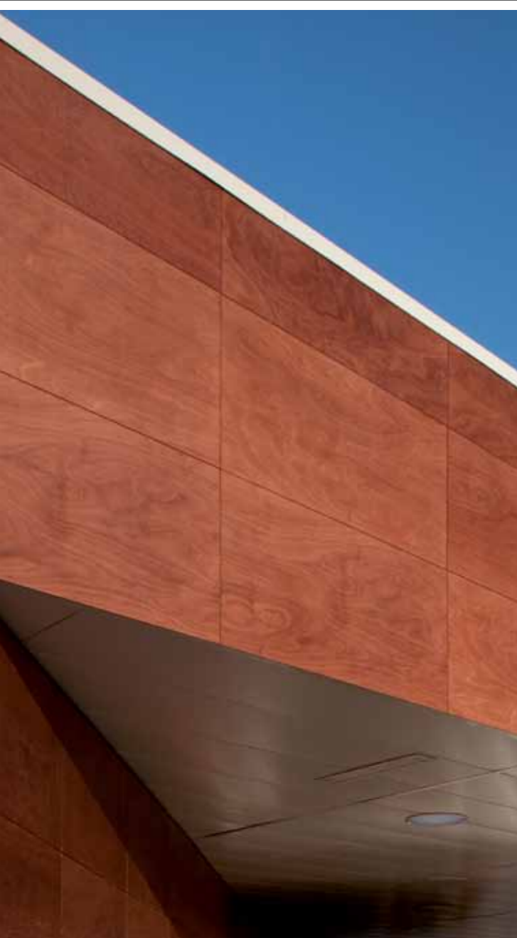
WALLS: VISIBLE FIXINGS
