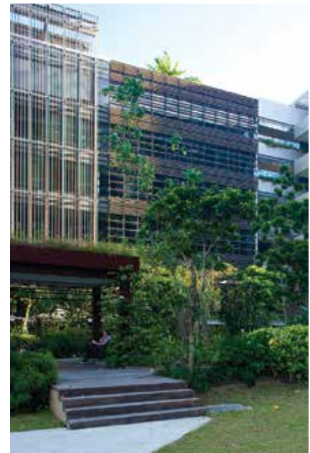
Above: The Khoo Teck Puat Hospital in Singapore by RMJM Architects uses fresh air and sunlight to increase thermal comfort. Image © Jui-Yong Sim/Flickr.
