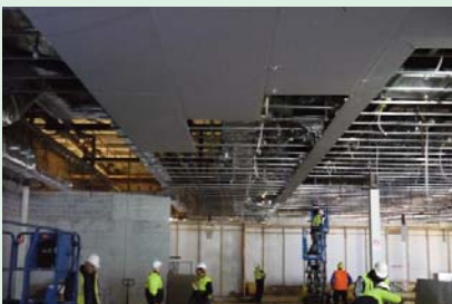
Studco concealed ceiling system engineered to provide a flexible and secure ceiling system.
