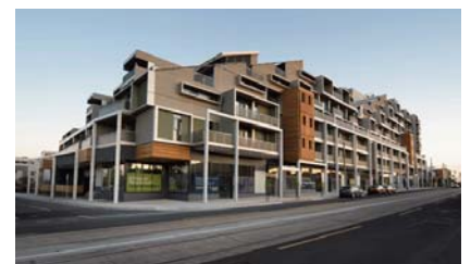
High rise apartments (nearly 200 actually!) constructed from stacked prefab modules.
