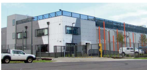
Factory-built, modular two-storey office complex consisting of 14 stacked modules.
