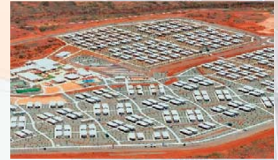
Mining town accommodation for more than 800 workers in Australia's Pilbara region.
