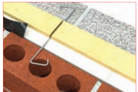
Wall tie sloping outward Sloping wall tie in pre-formed slot
