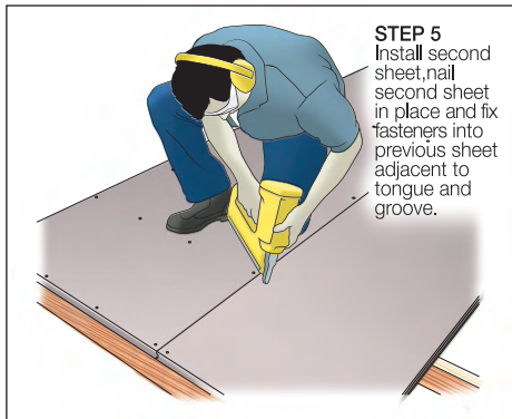
FIGURE 10 NAILING 2ND SHEET
