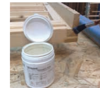
Teknoseal 4000 applied by brush to exposed end grain prior to factory finishing
