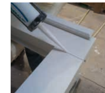
Applying Teknoseal 4001 to vulnerable v joints by cartridge gun
