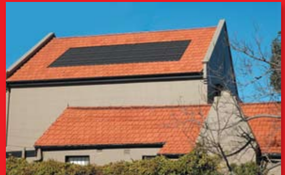
2kw solar roof approx.
