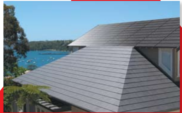
3kw solar roof approx.
