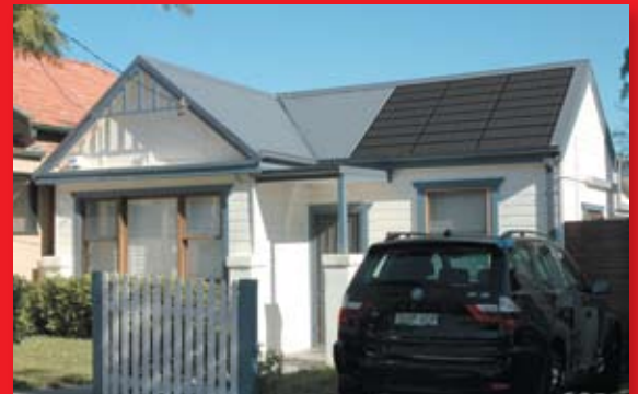
1kw solar roof approx.
