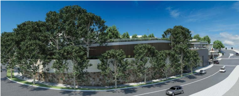
J Rosenthal Avenue Street and Planted Terrace We propose a wide verge, typical of Lane Cove, on Rosenthal Avenue around the outside of the Park with a generous footpath and native street trees with plenty of room to grow. The north-western wall of the development steps back to accommodate a 'garden terrace' with a second row of native trees and shrubs. This will provide a connection between the tree canopy at street level and the parkland above, softening the appearance of the development from adjoining residential areas. The footpath will provide access into and around the site for local residents.
