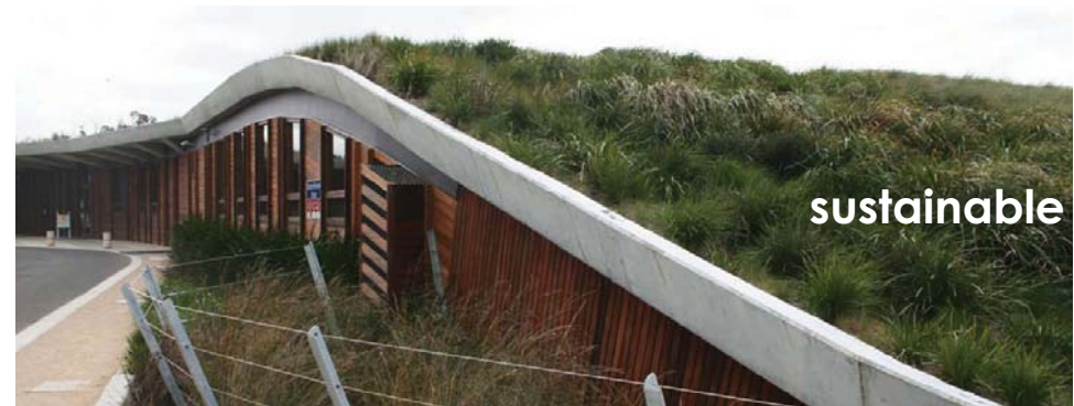
Green Roof, Queenscliff Photo: Arterra
