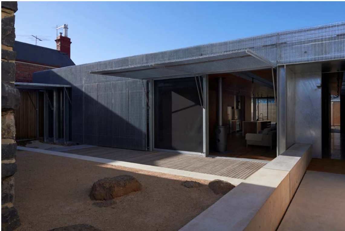
Edward Street House in Brunswick by Sean Godsell Architects
