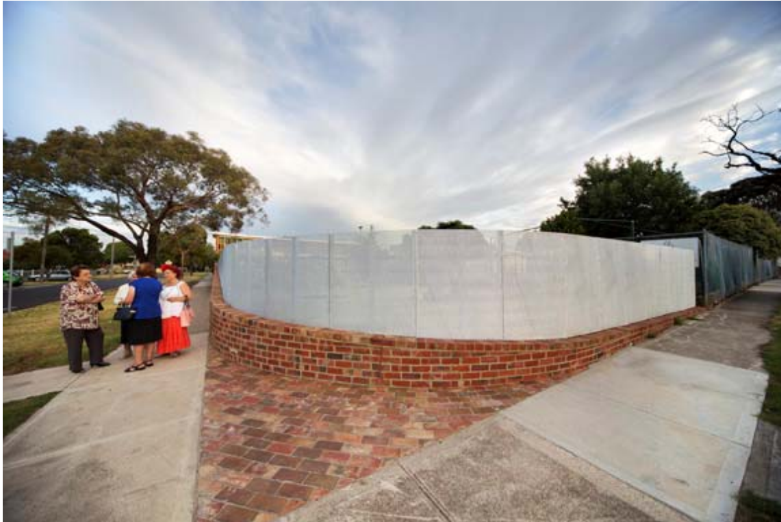
St Bernard's Parish Fence in Coburg East by Harrison and White with Paul Coffey Architects Photograph by Ben Hosking
