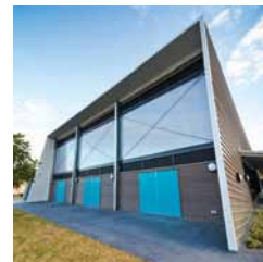
Low pitch roofing
