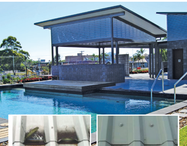
Standard plastisol on hot dip galvanised steel substrate roof after 7 years.
