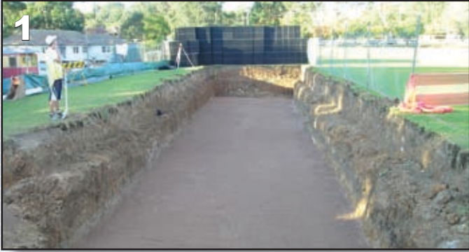
Excavation and Leveling.
