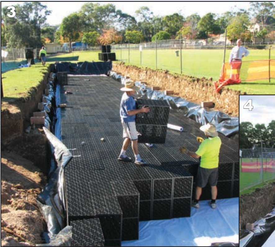
Installing Flo-Tank ® modules.
