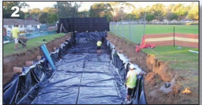
Installing Liner for Water Retention.
