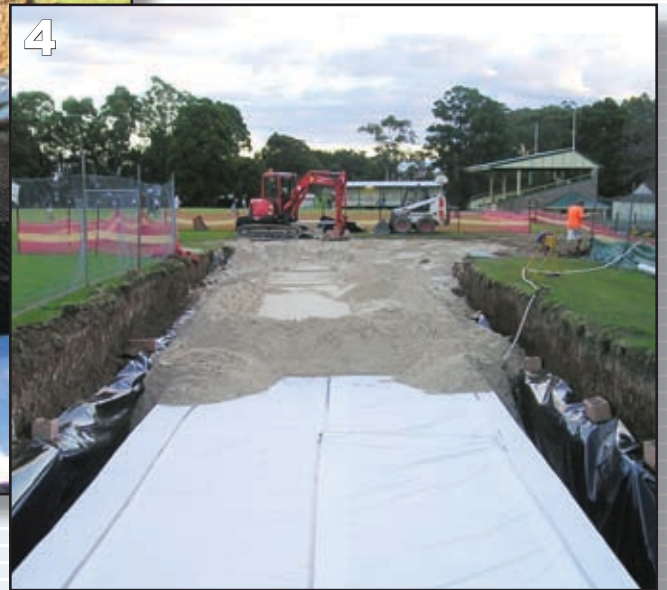
Backfilling with washed river sand.
