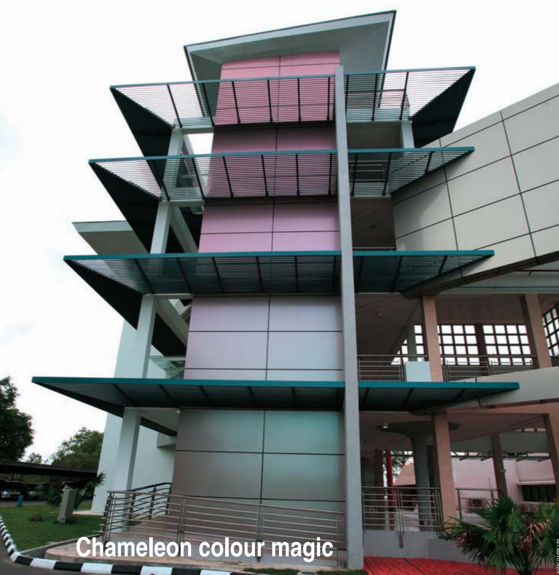
(From top to bottom) Alucobond Spectra Colours can give different colour effects depending on the angle of view.
