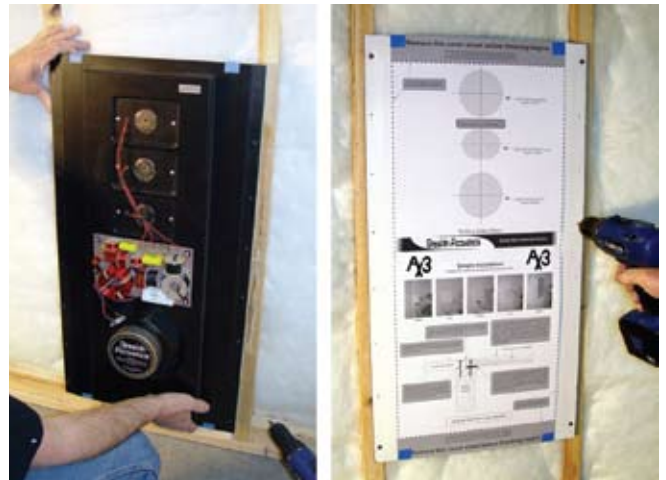
AX3 Speaker being installed - rear and front view
