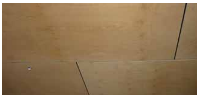
PremierWood in ceiling application
