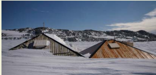
Mawson's Hut (1911 Antarctic Expedition) used Nordic Whitewood surviving the worlds harshest climatic conditions, testament to its strength and durability. Mawson's Hut Foundation heritage restoration 2006.
