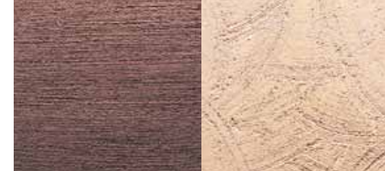
Broom Finish Trowel Finish
