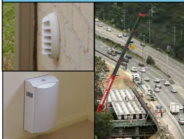
The Aeropac® ventilator has recently been installed as part of the Lane Cove Tunnel Project, Sydney, in surrounding dwellings.
