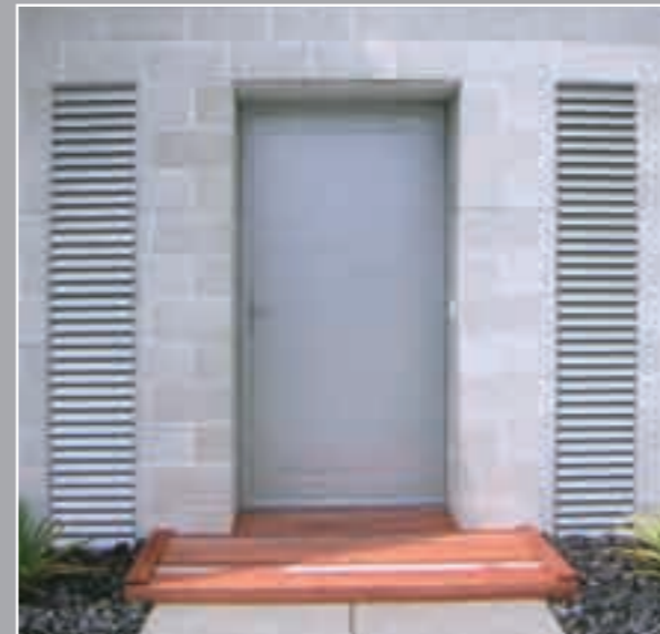
Louvre panels end fixed either side of entry door
