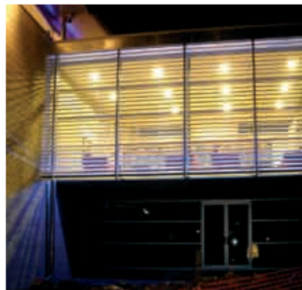
Motorised panels, 120 Airfoils
