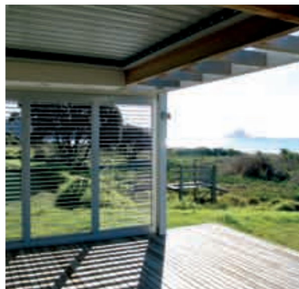
Single panel door viewed from inside with opening roof over
