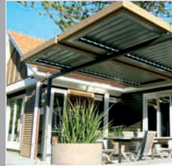
Twin opening roofs, cantilevered timber beams
