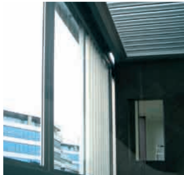
Sliding 180 Airfoil louvre panel, opening roof over
