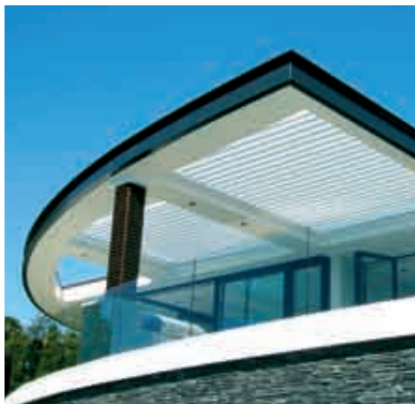
Opening roofs in cantilevered curved steel frame
