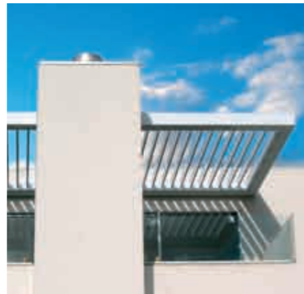
Large single panel opening roof in steel cantilevered frames
