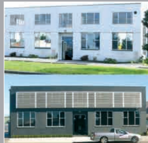
End fixed louvres, transforming the renovation
