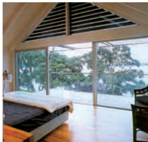
Pivoting panels of 120 Airfoils over deck, fixed triangular top panels
