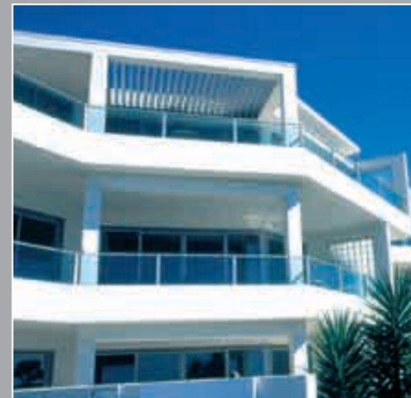
Opening roofs within plastered columns
