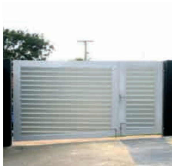
Pedestrian and vehicle gate on sloping driveway
