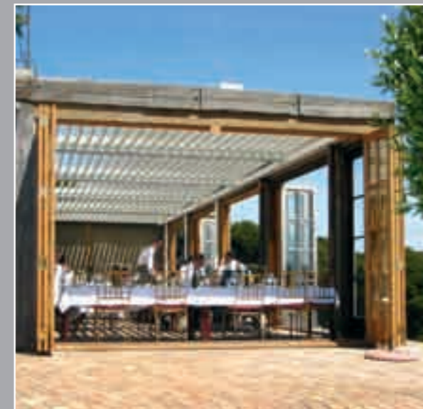
Multi panel opening roof in old timber beams
