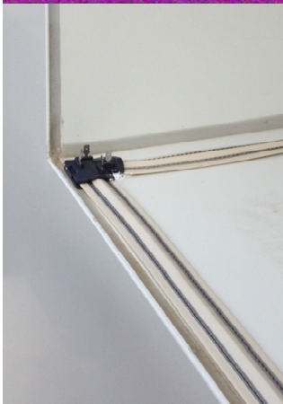
Neat corner fixings
