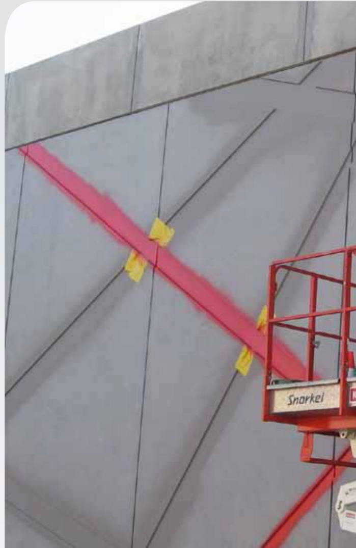
A highway acoustic barrier being coated in our Fluoropolymer
