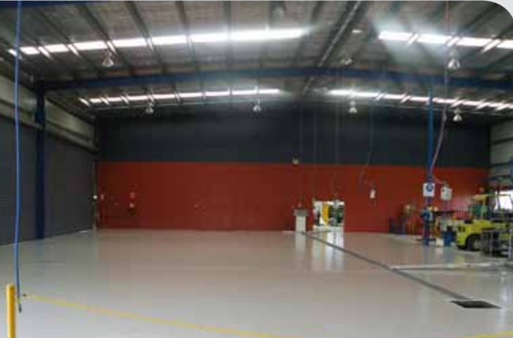
Anti-slip is essential for wash-down areas with falls to drains
