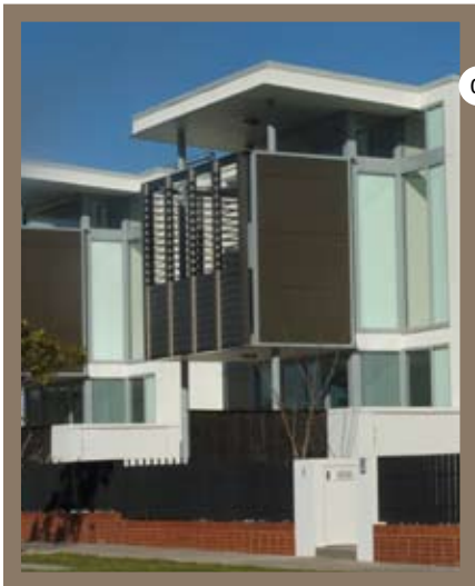
01. V2000 152mm toughened glass Louvre Blade used here to complement this office's contemporary design.
