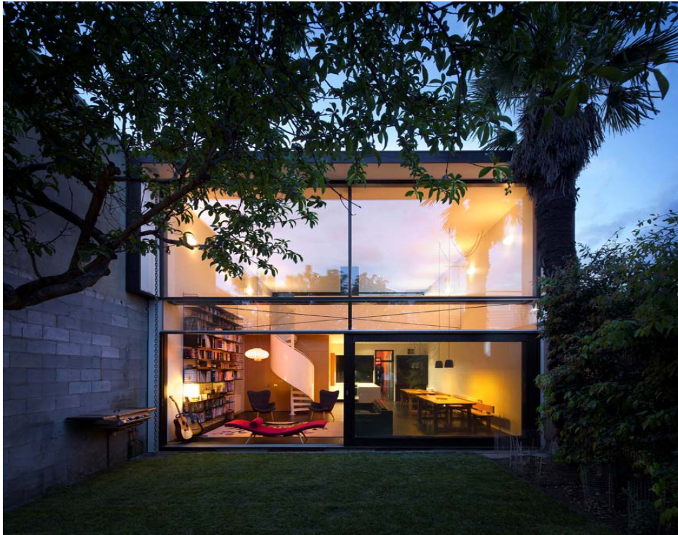
miller street in Richmond by three c architects
