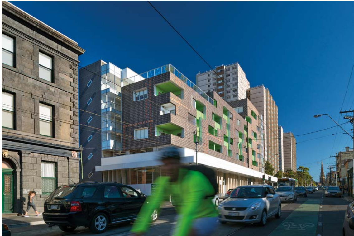
Atherton Gardens Social Housing and HUB Development in Fitzroy by McCabe Architects and Bird de la Coeur Architects Photograph by John Gollings
