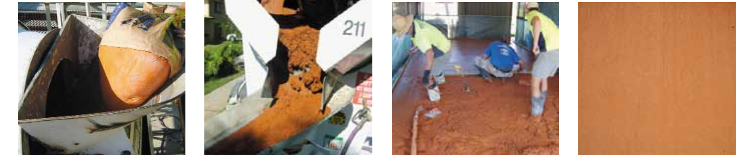
1 Preformulated bags of CCS pigment concentrates are added to the concrete truck at the predesignated rate of one bag (or sometimes two, depending on the colour) per cubic metre.
