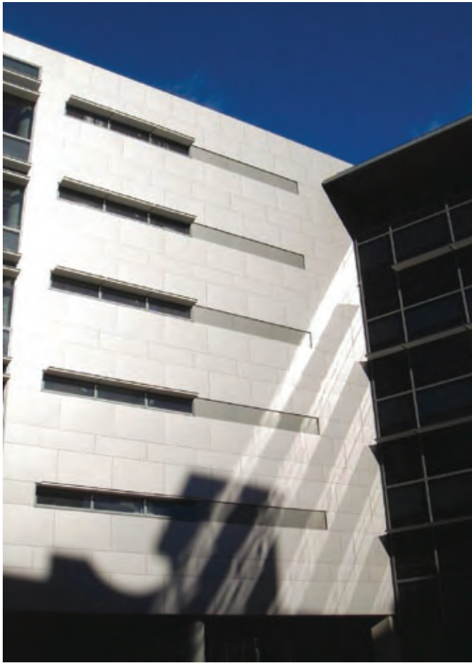
Fairfax Media Offices - Sydney, NSW Architects: HPA Architects
