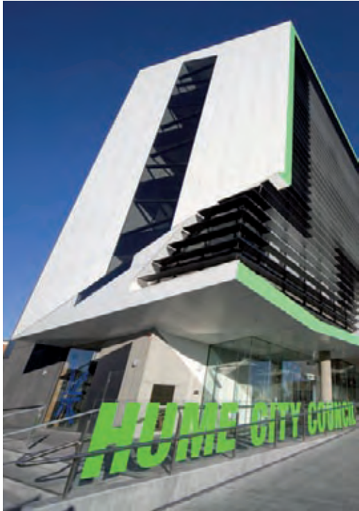
Hume City Council Building - Hume, Vic Architects: Lyons Architects
