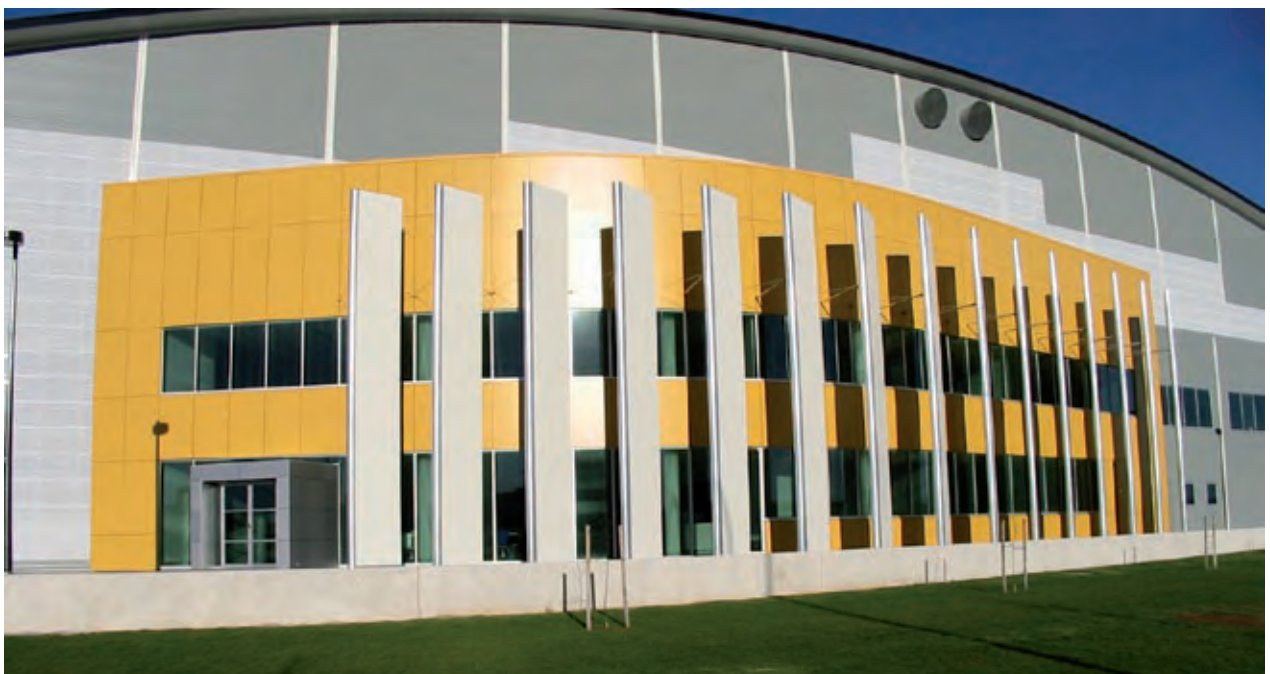
Qantas Hangar - Canberra, ACT Architects: Daryl Jackson Alastair Swayn P/L
