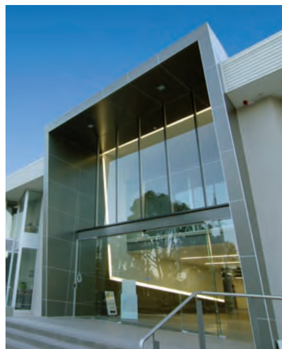
smartfix® Head Office - Canberra, ACT Architects: Turco Hunter Architects
