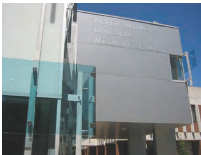
Australian National University, Medical School - Canberra, ACT Architects: May Russell Architects
