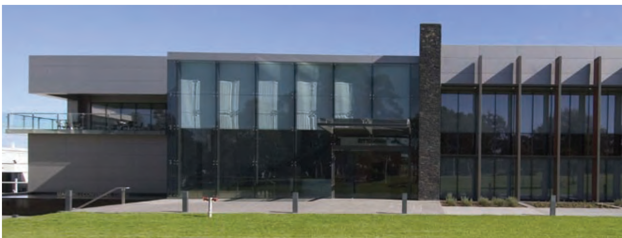
Pfizer Learning / Conference Centre - West Ryde, NSW Architects: Project Control Group
