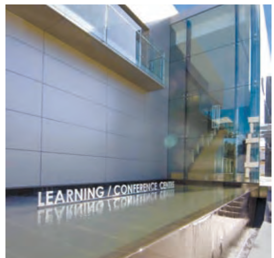
Pfizer Learning / Conference Centre - West Ryde, NSW Architects: Project Control Group
