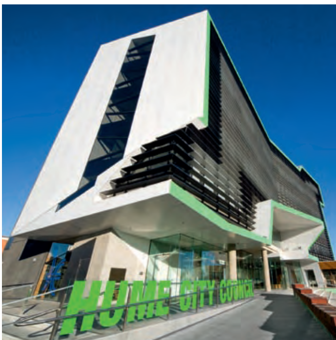
Hume City Council Building - Hume, Vic Architects: Lyons Architects
