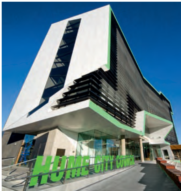
Hume City Council Building - Hume, Vic Architects: Lyons Architects
