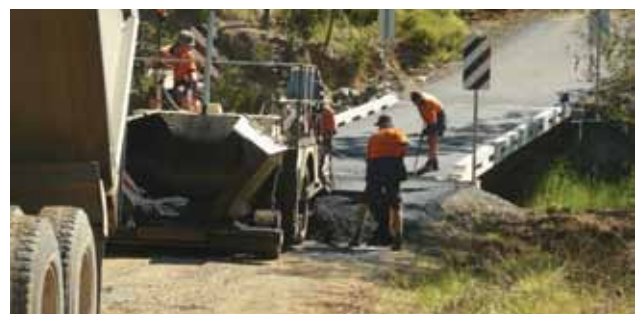
Road surface work on BridgeWood
