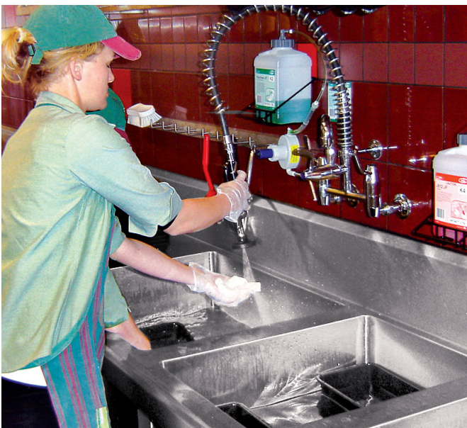
A #TF83WJP-W - CP Ezy-Wash Wall Mounted Exposed Mixing Pre-Rinse Unit Type 83W, 15BSP Female Inlets with Pot Filler (Modified) (Photo courtesy of Woolworths Redcliffe, QLD).
