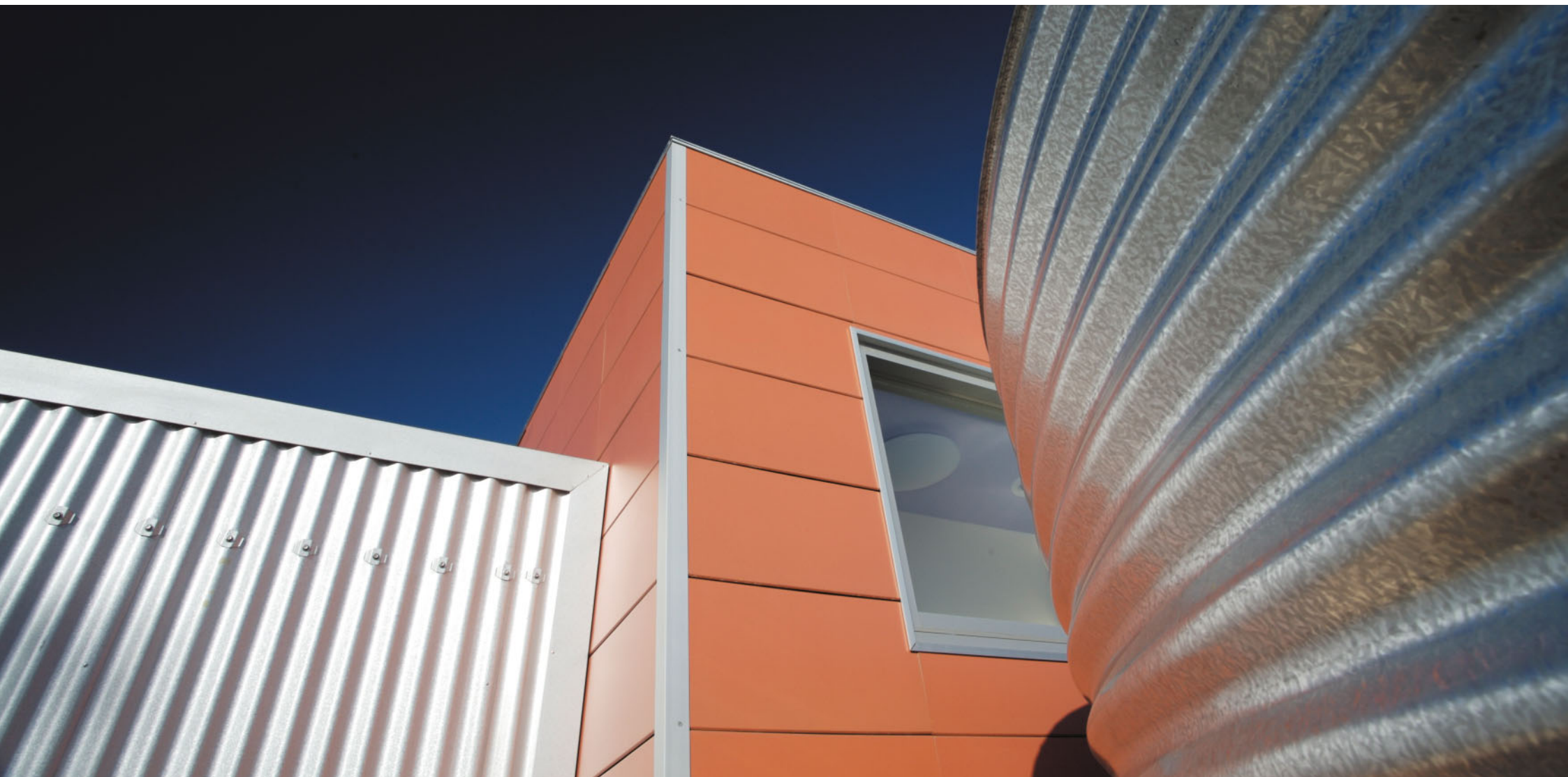
PROJECT: McKinnon Primary School . McKinnon . Victoria ARCHITECT: Kneeler Design
